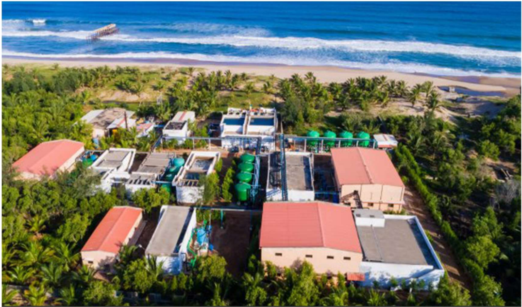
Fig. 2.4 Desalination plant in the Hetero Premises
