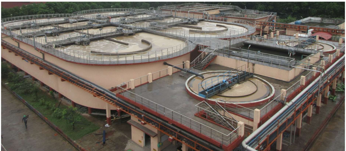
Fig.2.9: Biological system for LTDS & Condensate of MEE & ATFD
