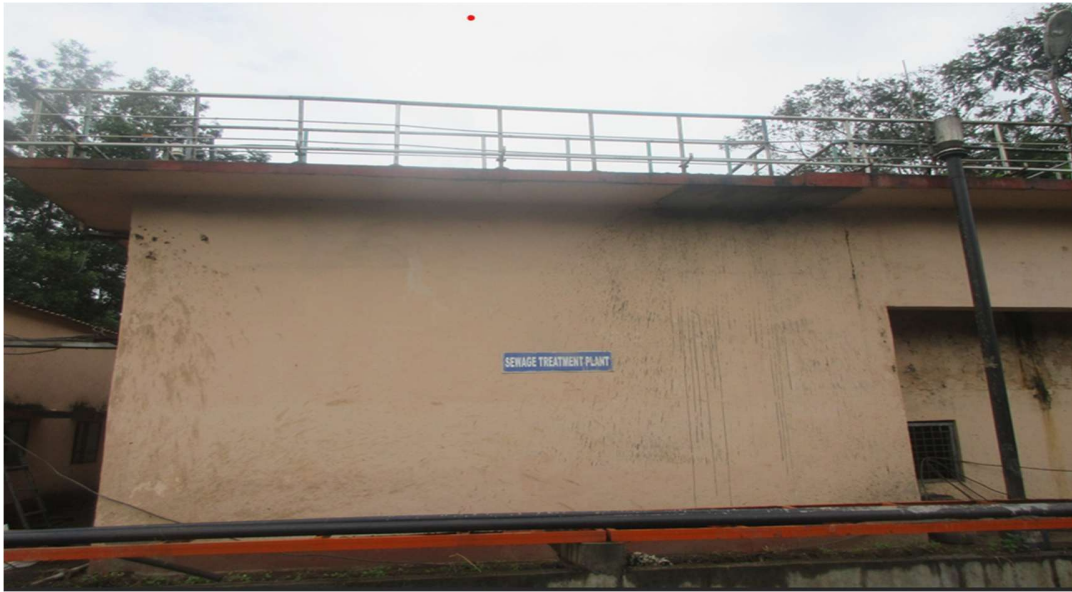
Fig.2.6: Sewage Treatment Plant (STP)
